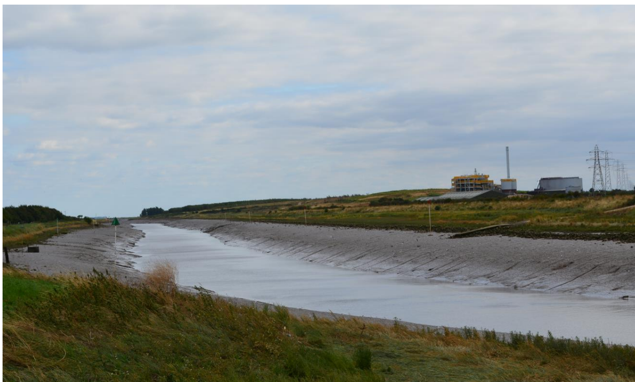
Plate 11 The Haven Facing South (with the Boston Biomass UK No.3 Ltd Gasification Plant on the Right). Photographs Taken 16th August 2018.
